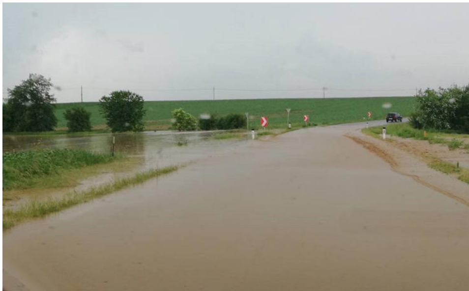
Figure 5.2: Flooded road between Weitersfeld and Prutzendorf during the heavy rainfall event on the 1st of June 2018. (Photo: Österreicher 2018)
