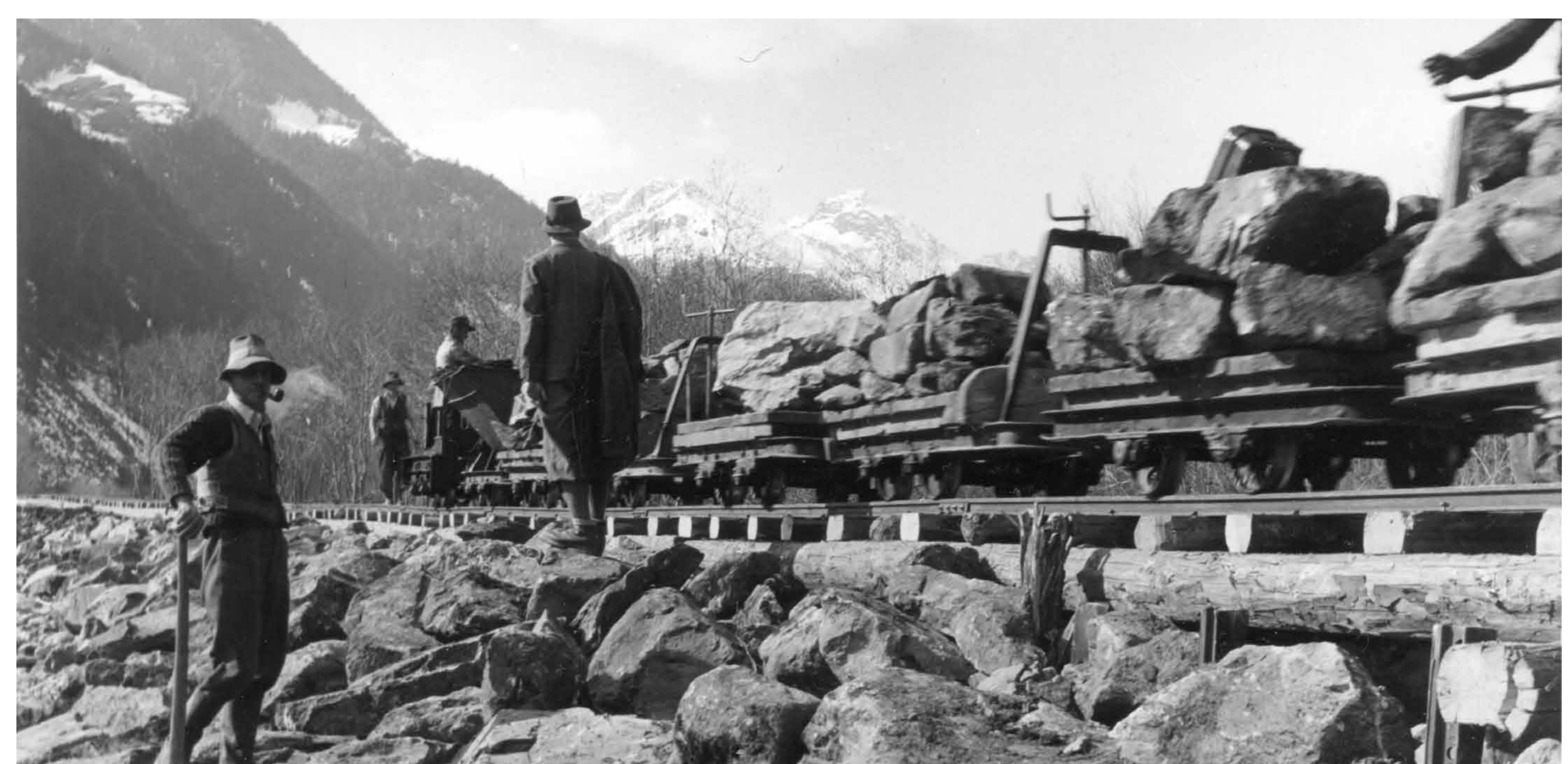
Transport of hydraulic construction stones with diesel locomotive on light railway
