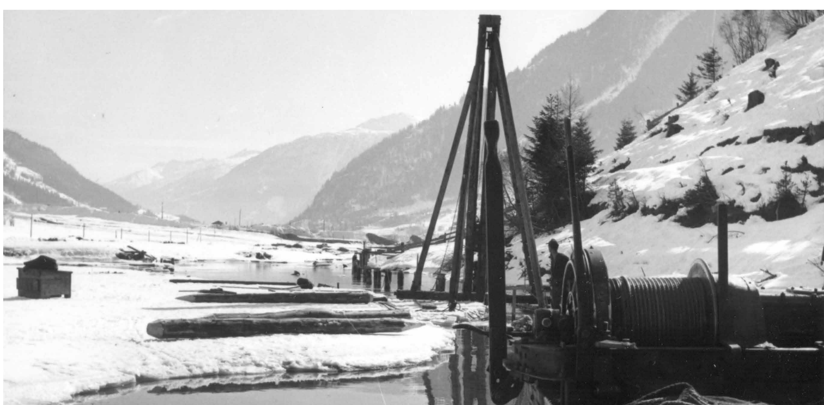
Moving wooden pilots using a diesel pile driver
