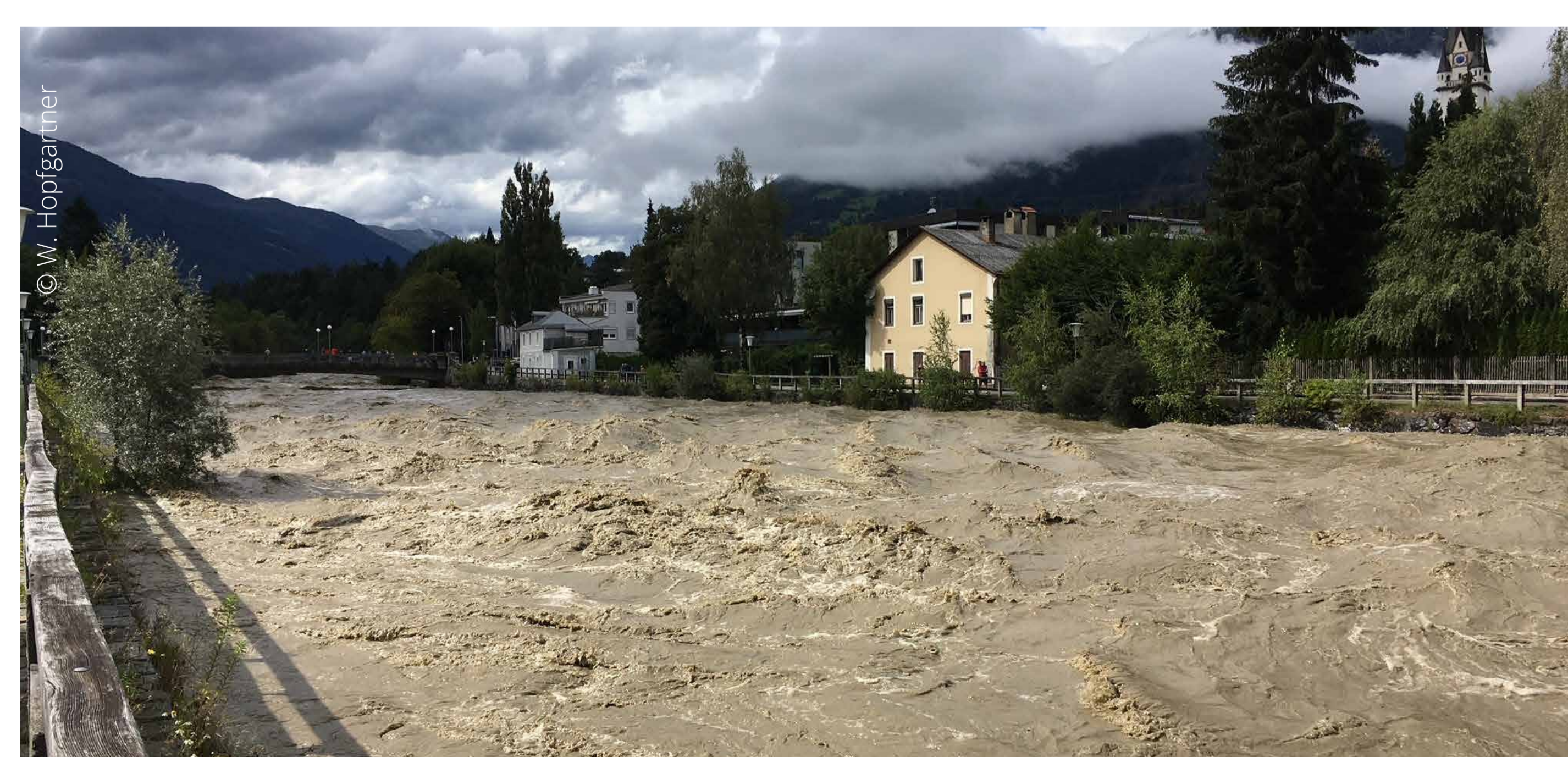
Lienz August 2020, the widening upstream is effective, the extreme flood event has no consequences for the town.
