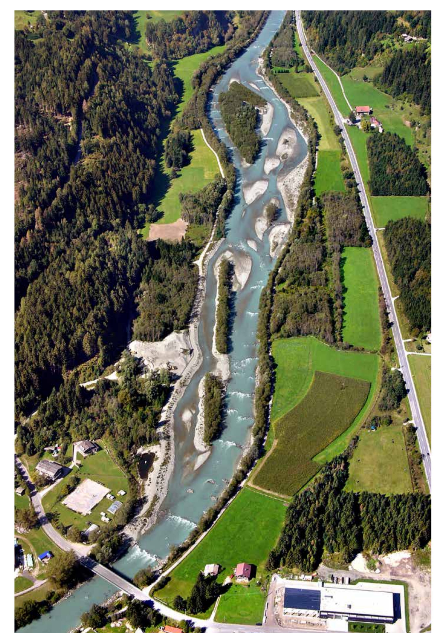
Expansion of Weierburg gravel basin, Ainet: Length 650 m
