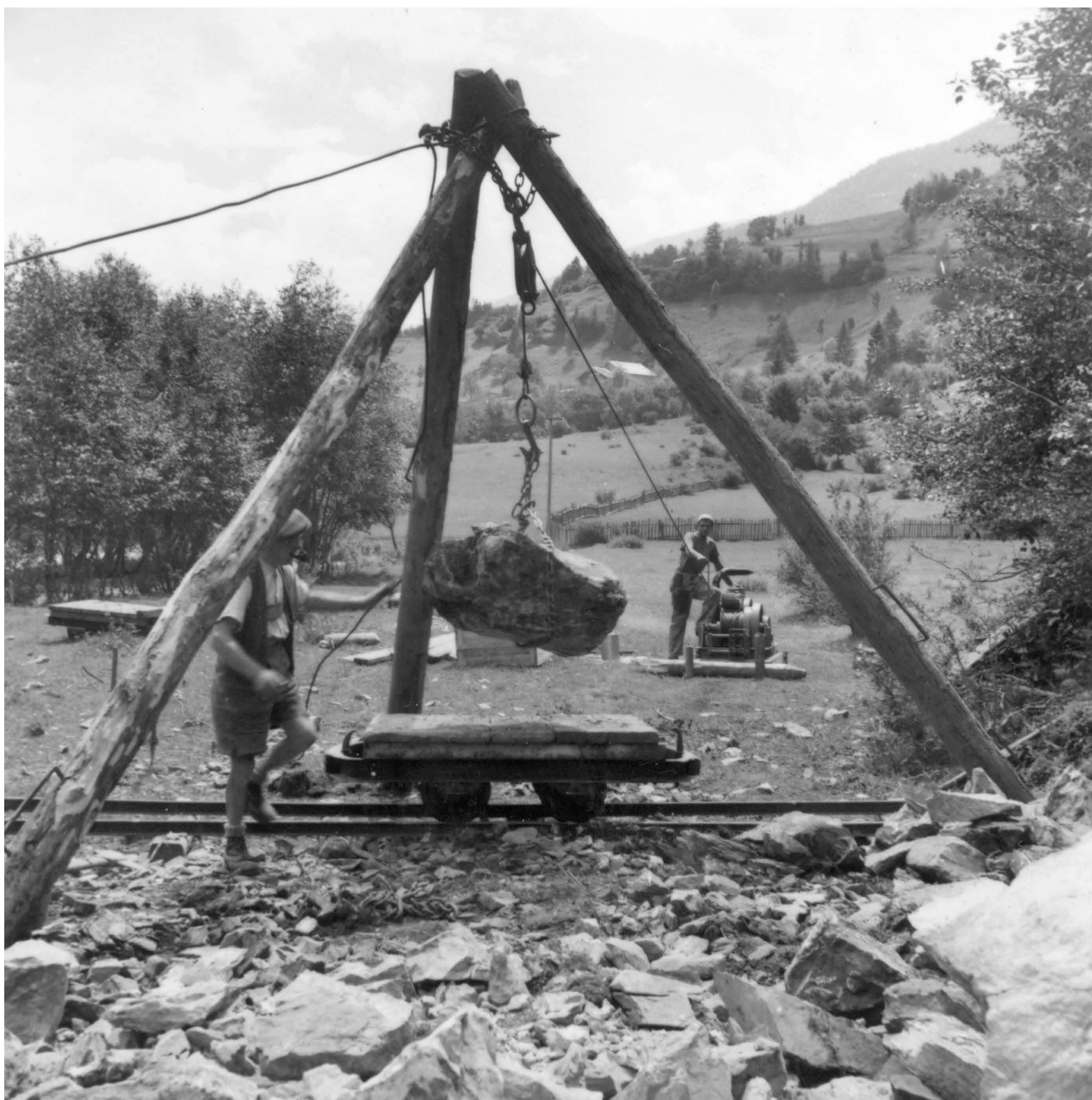
Loading river blocks with tripod scaffolding and cable winch
