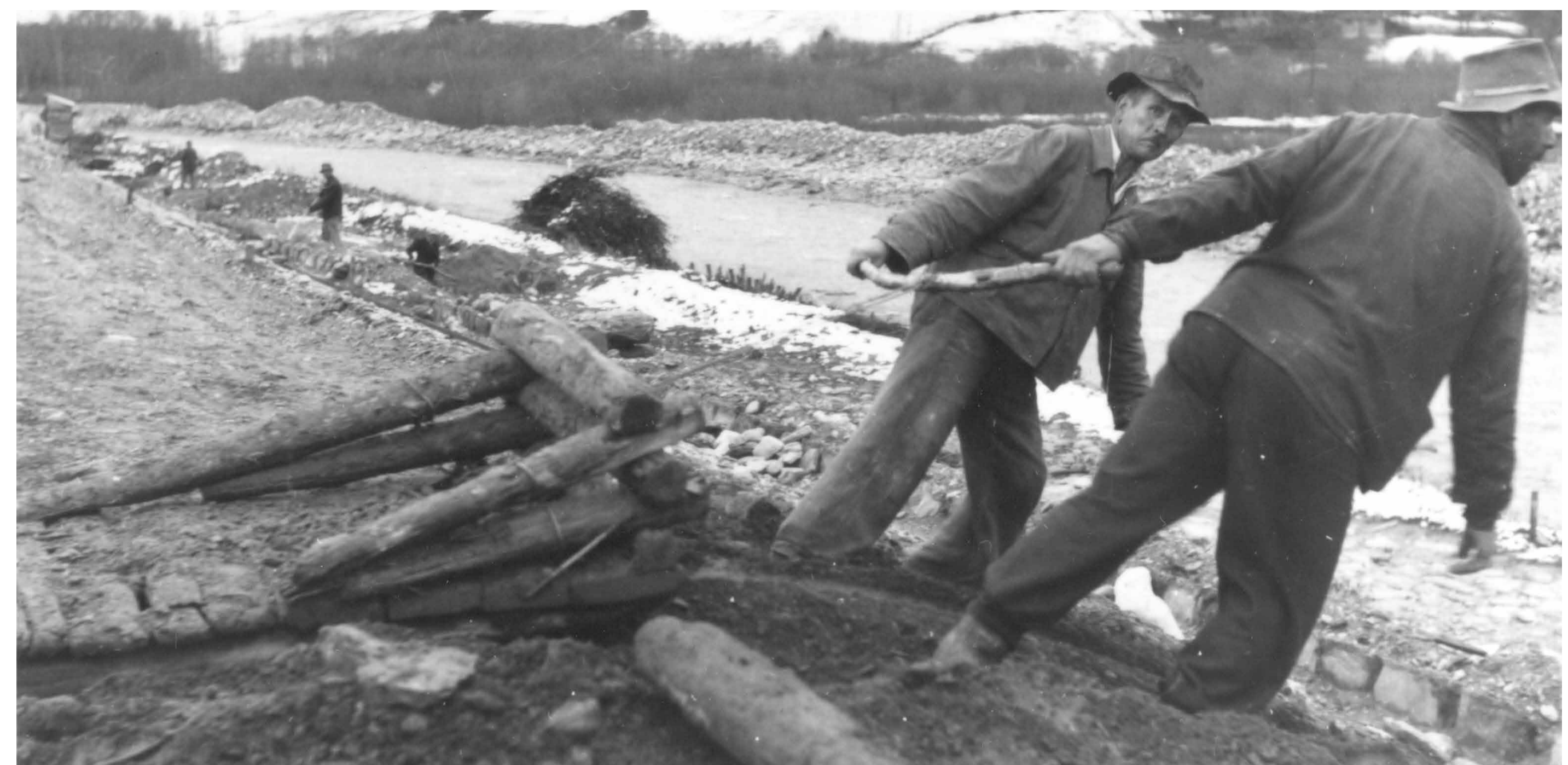
Clearing debris landings using wooden sledges and cable winch
