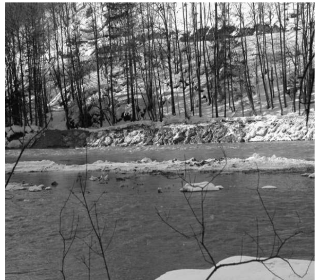
Fig. 4: Shore stabilisation: Rough stone layering, coins under water level
